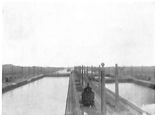
Section of Gatun Lock, Panama Canal.
