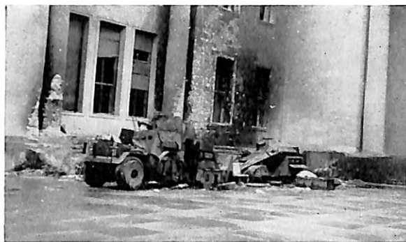
The Inner Courtyard of the Chancellery.
