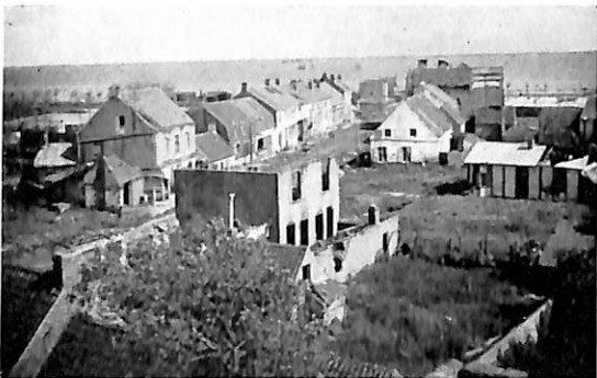
Flooded area south of Ghyvelde, looking S.W. from forward O.P.
