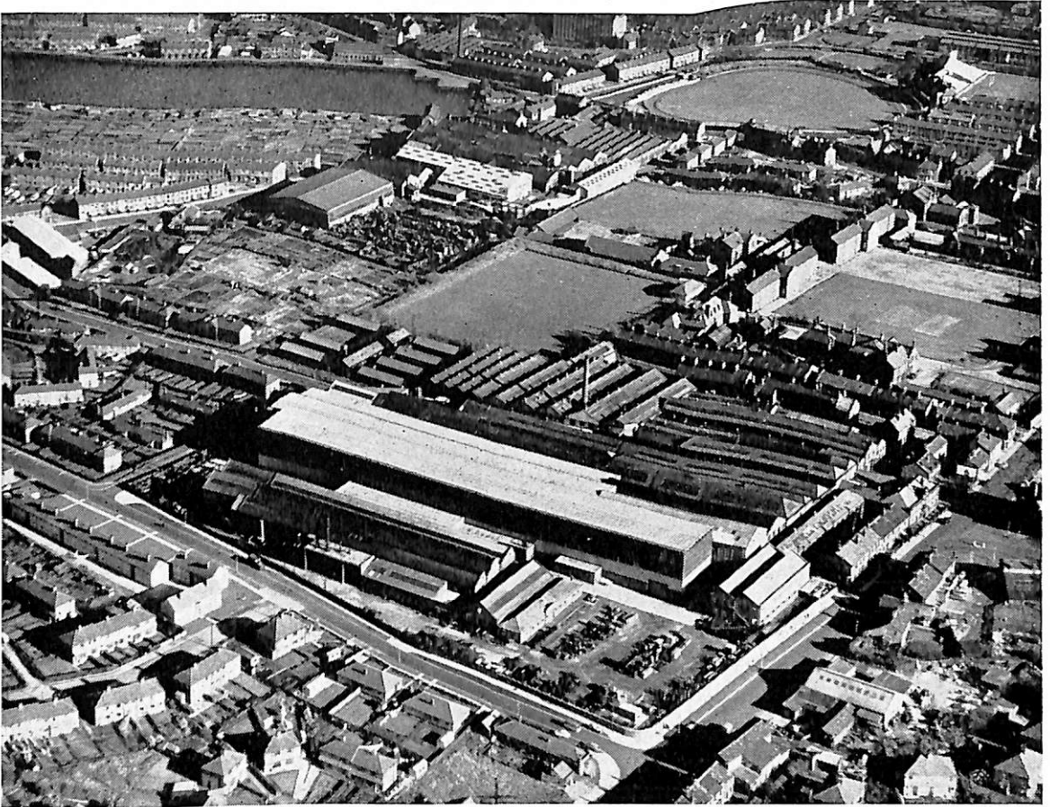
A recent aerial view showing the Asquith works, with Wellesley Barracks to the right of the picture
