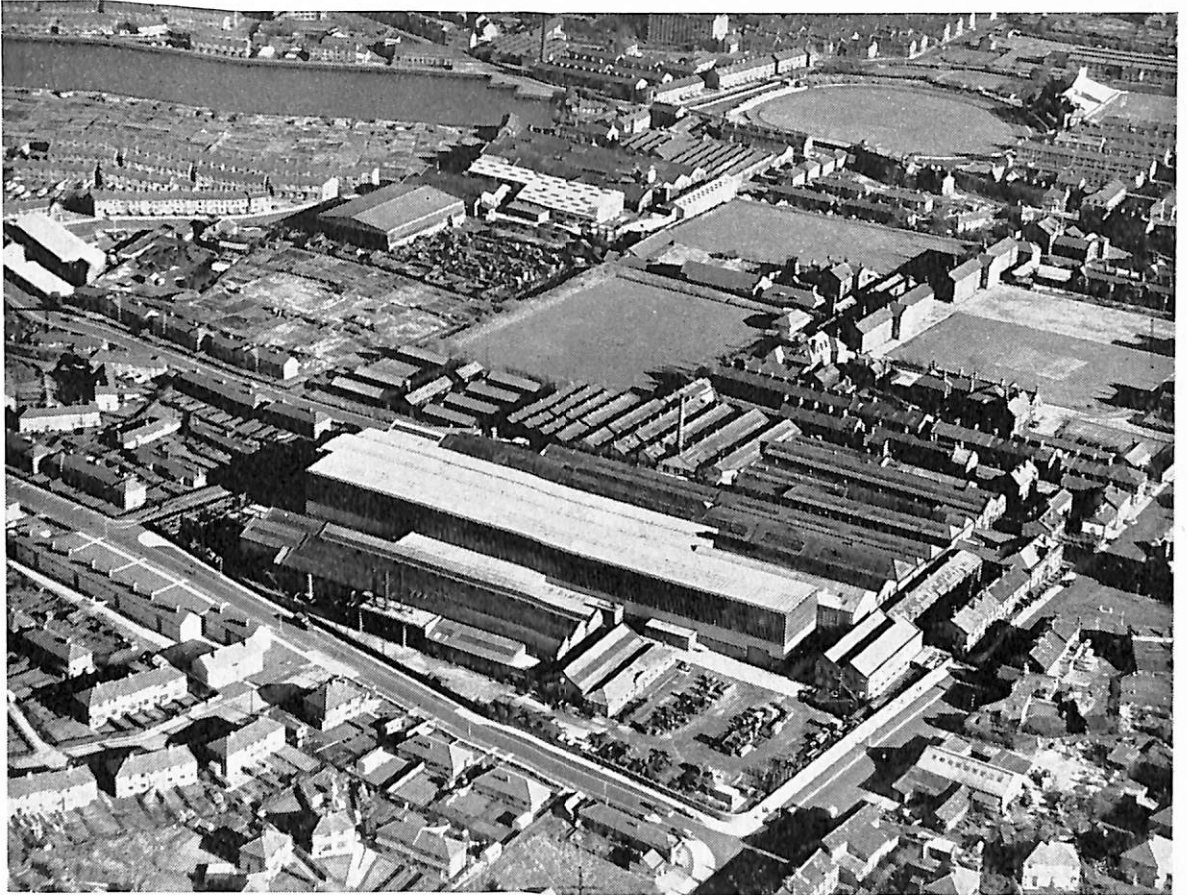
A recent aerial view showing the Asquith works, with Wellesley Barracks to the right of the picture
