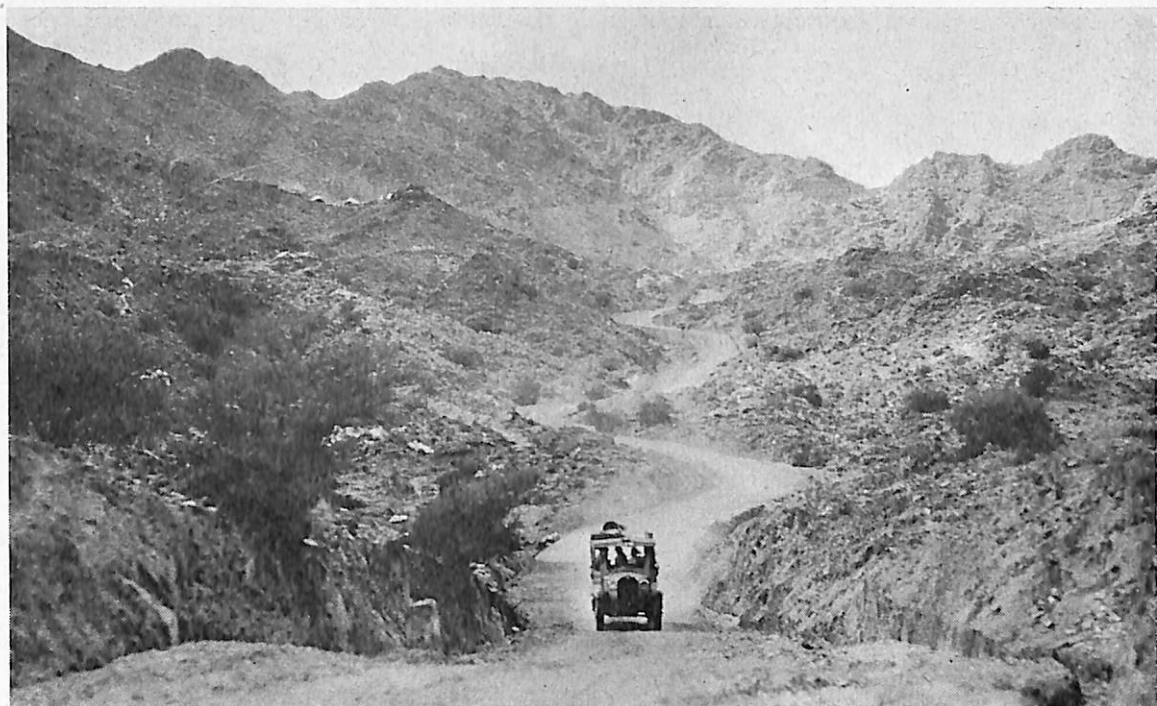
Road between Subhan Khwar & Kilagai
