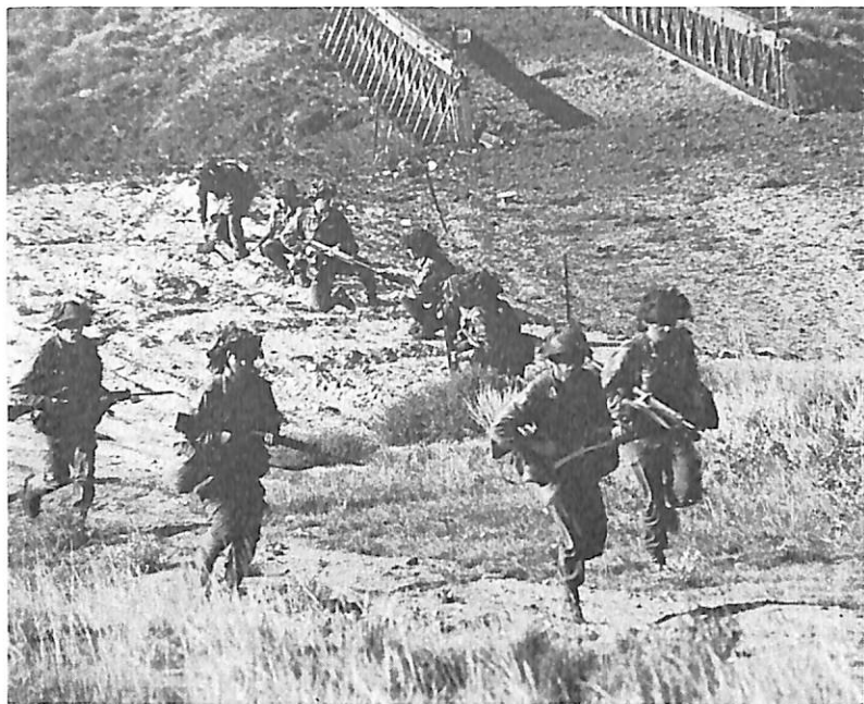
Training in Canada 9 Platoon withdrawing after a Bridge Demolition
