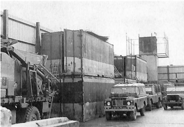
From Crossmaglen to Catterick (1) Somme Company accommodation at Crossmaglen for 4 days!
