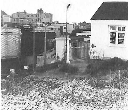
Corunna Company's Project Before
