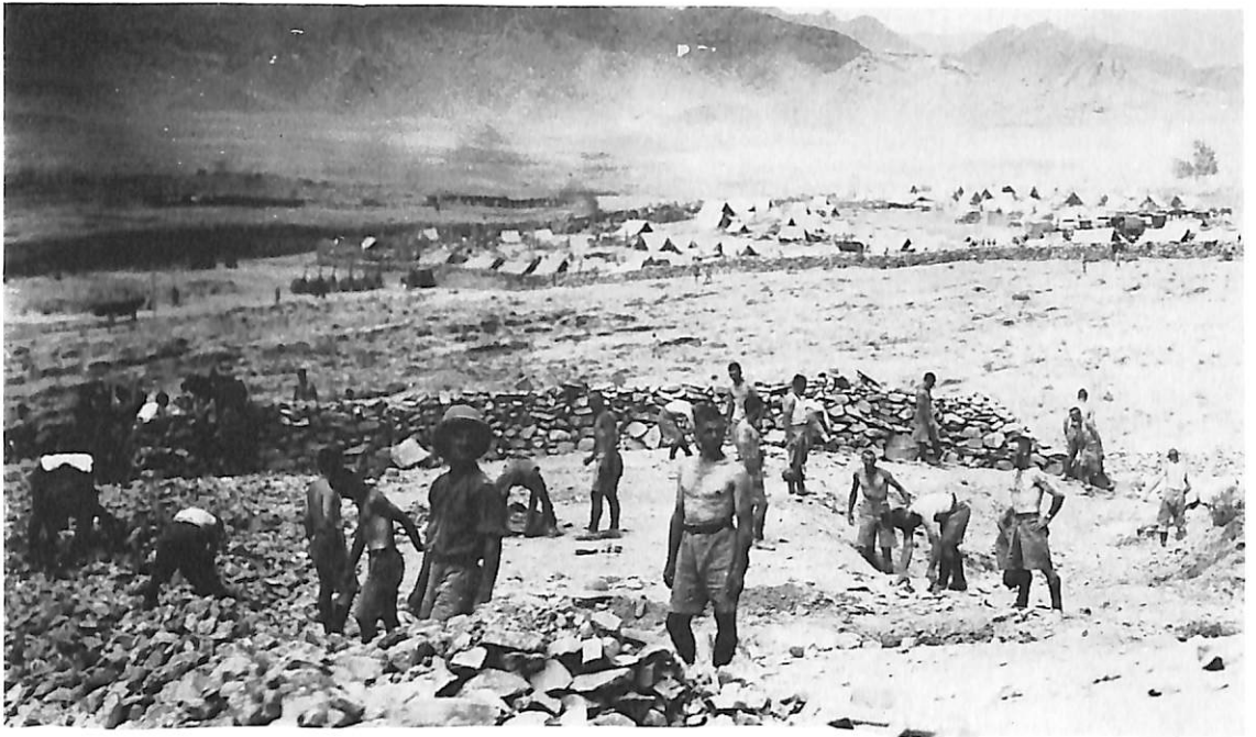
The Nowshera Brigade Members of the 2nd Battalion building defensive walls against night snipers.
