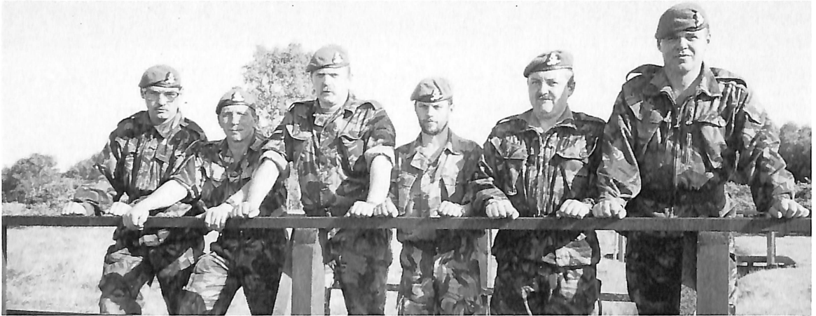
Left to right: Private Turner, Sergeant Wasden, Colour Sergeant Moore, Sergeant Stowe, Corporal Ackroyd, Private Evans. Assault Pioneers on the vehicle bridge they helped to build on Strensall Ranges for Range Warden's vehicles. May 1998.
