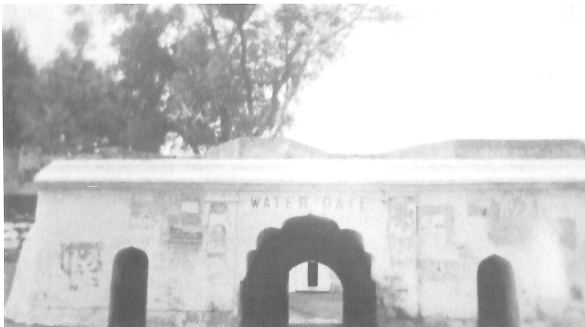
The Water Gate
