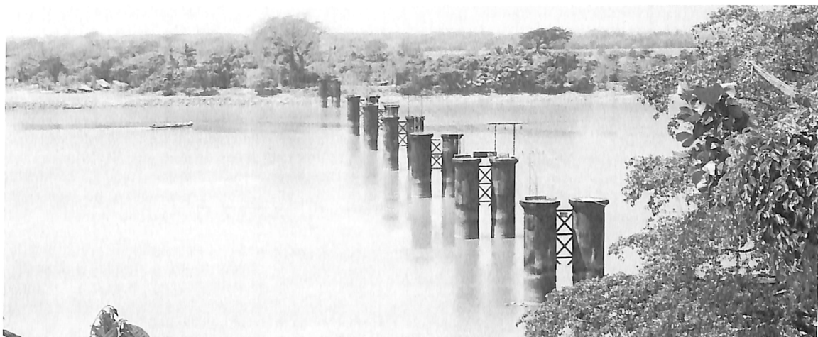
Piers of Sittang Bridge from rail level, south east corner.
