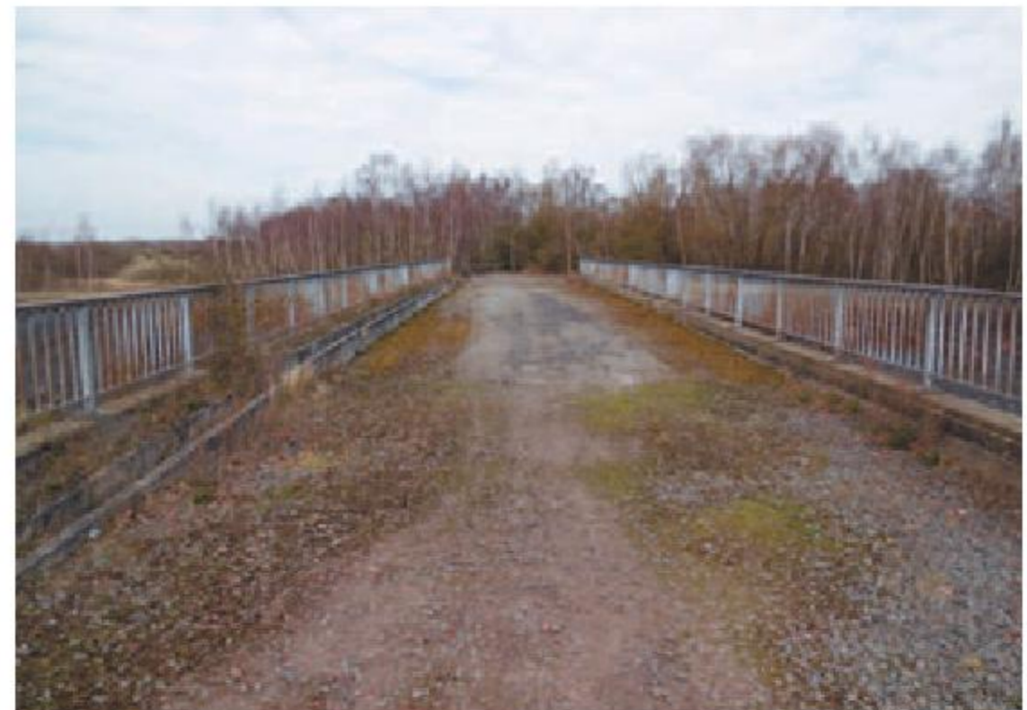
The old railway bridge, defended by a company of 1 RWK and the machine gun section of 2 DWR
